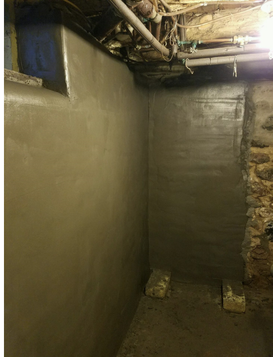
Example Xypex Megamix II over concentrate installed on stone wall.
