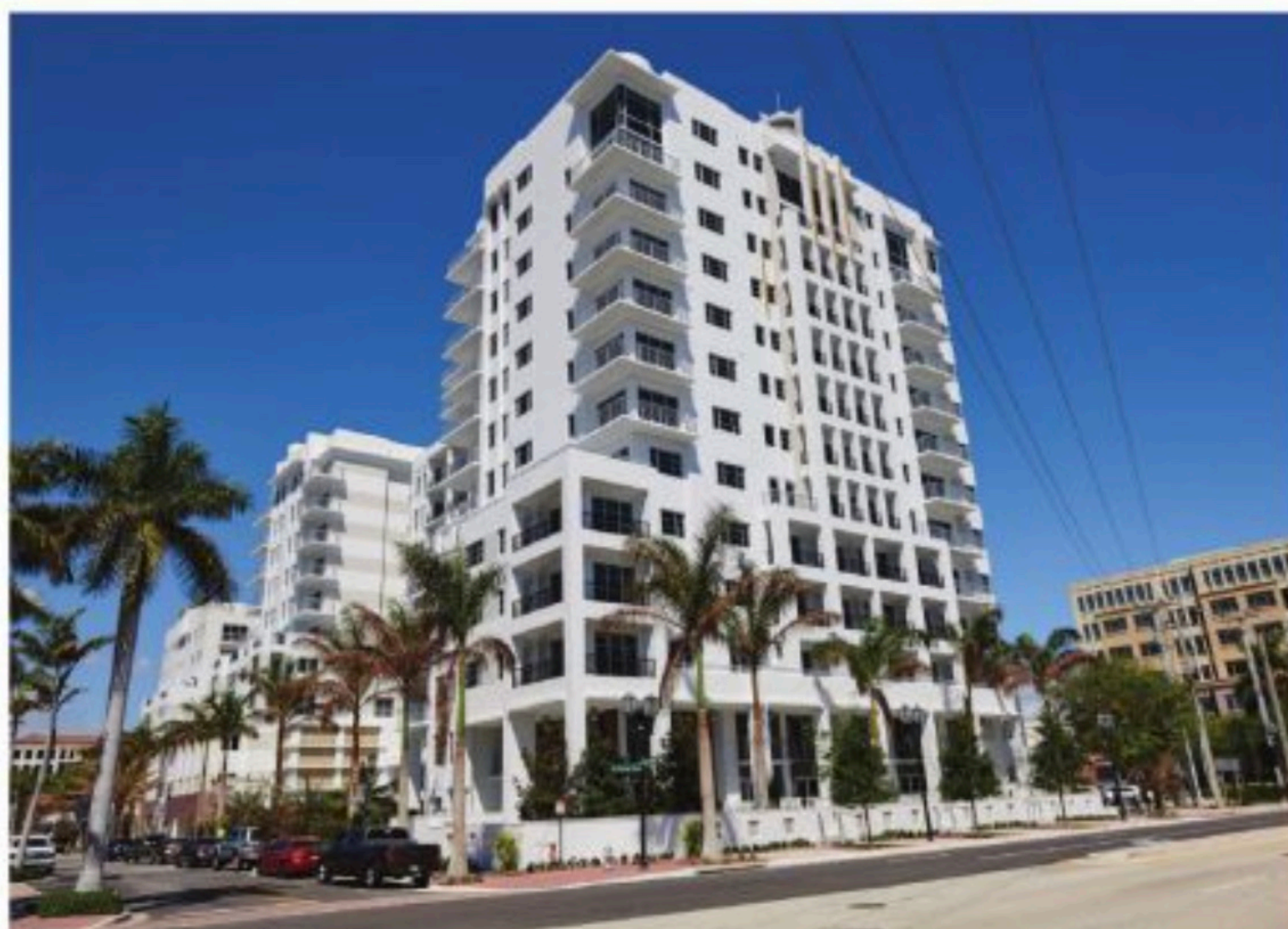
Tower 155 in Boca Raton, Florida, is a 14-story condo complex featuring 170 luxury units. The foundation is constructed 6 m (20 ft) below grade and has a two-level, below-grade parking garage. Crystalline admixture waterproofing was added to the 5199 m 3 (6800 cy) concrete used to pour the foundation slab, walls, swimming pool, and spa fountain.
