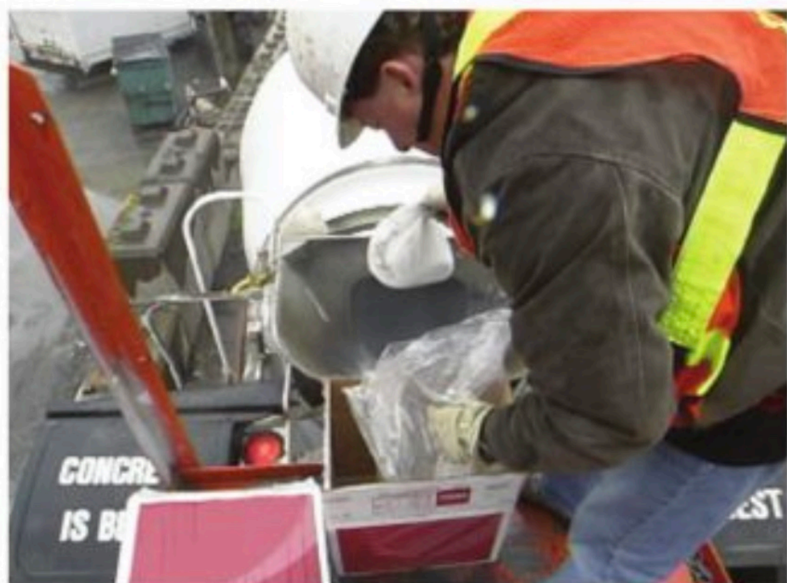
Crystalline waterproofing in water soluble bags is added to the back of a ready mix truck.
