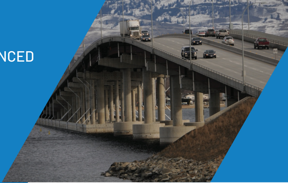
William R. Bennett Floating Bridge, Kelowna, Canada
