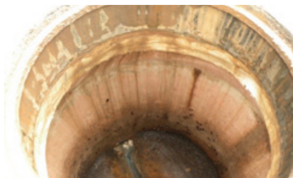
Terrebonne Parish manholes with crystalline admix show little deterioration after 10 years of service.
