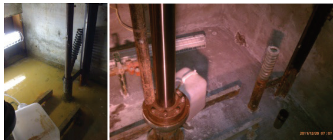
Images of elevator pit before and after application of crystalline waterproofing
