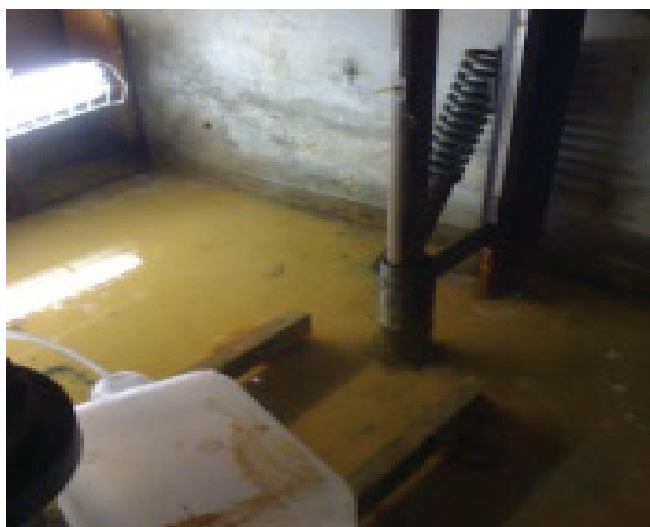
Water Ingress in Elevator Pit
