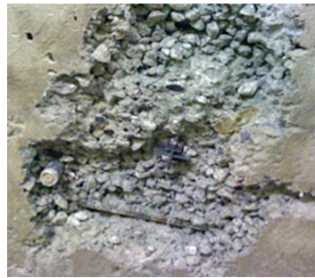
Construction defects (rock pockets, honeycombs & untreated tie holes)
