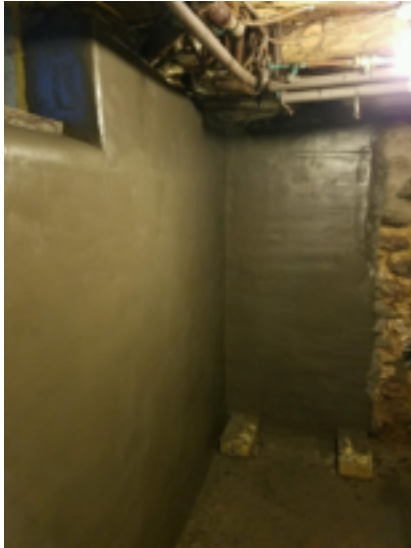
Example of Xypex Megamix II over Concentrate installed on stone wall
