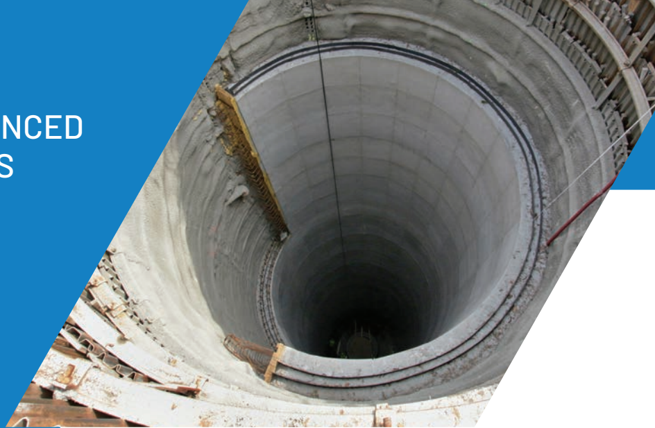
Prague Sewer Tunnels, Ďáblice, Prague, Czech Republic
