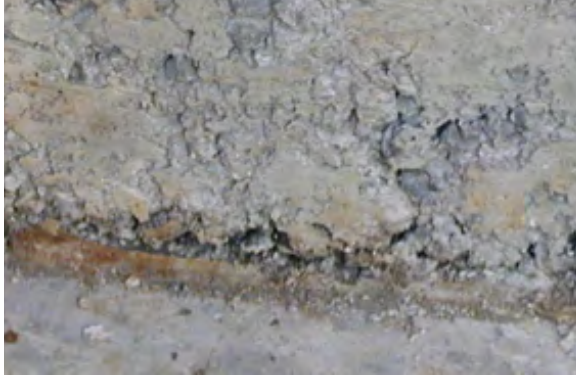
Example of Poor Wall to Slab Joint Consolidation
