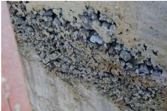
Examples of areas of poor concrete consolidation
