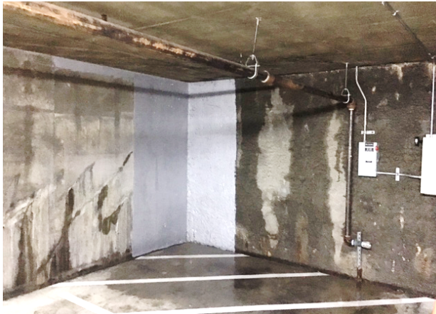
Examples of below grade structures that are leaking and in need of repair
