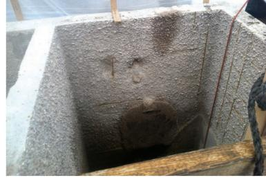
During a routine inspection, engineers noted that the surfaces of the concrete siphon chamber showed signs of significant deterioration from MIC, which is a direct result of  $H_2S$  gas.
