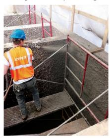
faces of the concrete siphon chamber showed signs of significant deterioration from microbial
