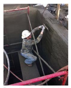
The crystalline waterproofing technology is non-toxic and contains no VOCs. This makes the crystalline material an ideal solution for applications in confined spaces.
