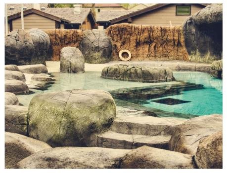
The new sea lion exhibit at the St. Louis Zoo features a shotcrete exterior made with a Xypex Concrete Waterproofing through Crystallization admixture to help prevent leakage of the habitat's salt water pools, underwater viewing areas, and an underwater walk-through tunnel.
