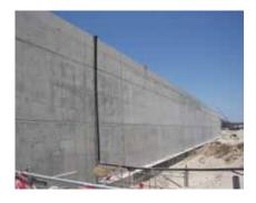
of the concrete and become a permanent part of the concrete mass... [and] resist water penetration against hydrostatic pressure." The crystalline chemistry delivers an integral waterproofing system without the exposure disadvantages (from tearing or detachment) presented by external barrier/membrane solutions. It also is generally less costly and more convenient than external barrier approaches.
