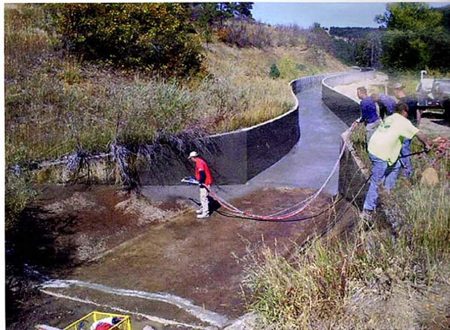
Application of Xypex Concentrate at flume opening.
