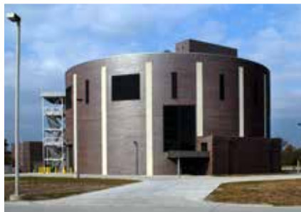
Fig 2 -- Lift station for the Lower Meramec Wastewater Treatment Plant pumps sewage from the four-mile long Baumgartner interceptor tunnel — located 200 feet underground—up to the water treatment plant at ground level.
