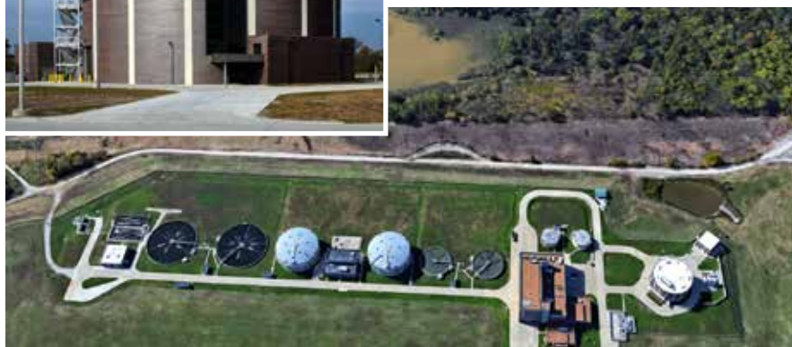
Fig 2 -- Lift station for the Lower Meramec Wastewater Treatment Plant pumps sewage from the four-mile long Baumgartner interceptor tunnel — located 200 feet underground—up to the water treatment plant at ground level.
