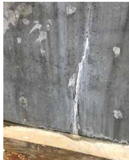
Fig 10 – BEFORE (left) – a hairline crack in the newly poured channel wall is actively leaking during hydrostatic testing. Efflorescence indicates Xypex crystalline growth has been activated by the presence of moisture. AFTER (right) – the same crack about a month later shows signs of crystal growth and has self-healed. Efflorescence can be brushed off if desired.
