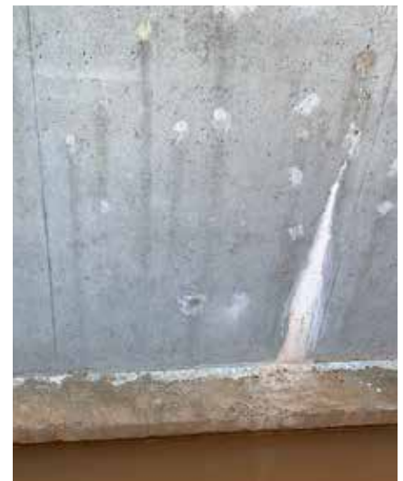
Fig 10 – BEFORE (left) – a hairline crack in the newly poured channel wall is actively leaking during hydrostatic testing. Efflorescence indicates Xypex crystalline growth has been activated by the presence of moisture. AFTER (right) – the same crack about a month later shows signs of crystal growth and has self-healed. Efflorescence can be brushed off if desired.
