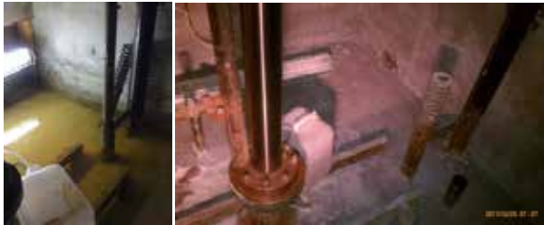
Images of elevator pit before and after application of crystalline waterproofing
