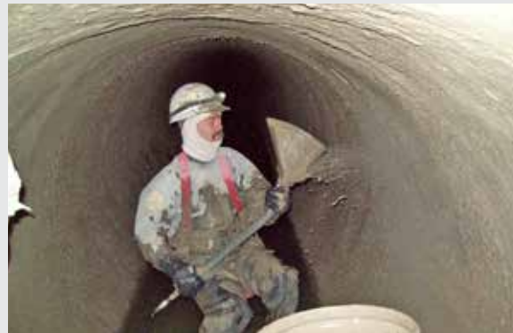
Xypex Concentrate followed by Xypex Megamix I is applied in second 8-hour closure.
