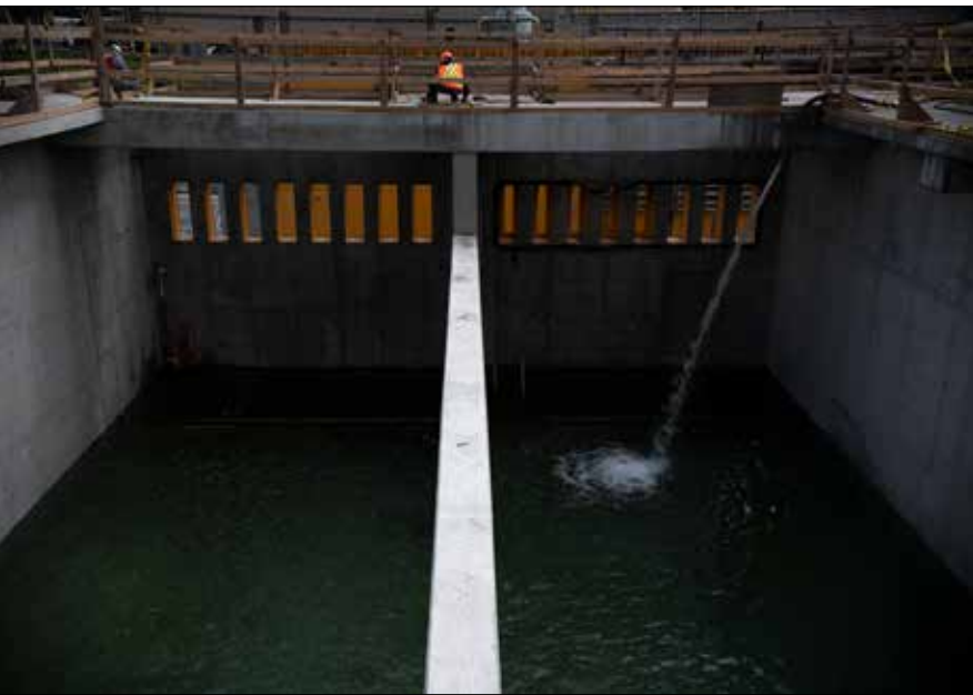
AGRU waterproofing in action
