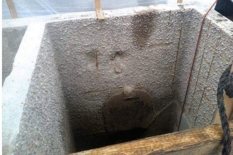
During a routine inspection, engineers noted that the surfaces of the concrete siphon chamber showed signs of significant deterioration from MIC, which is a direct result of H<sub>2</sub>S gas.
