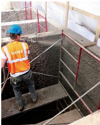
The contractor first blasted the concrete clean with high-pressure, water-based abrasive and then installed Xypex Megamix II resurfacing mortar to thicknesses ranging between 2 and 3 inches.
