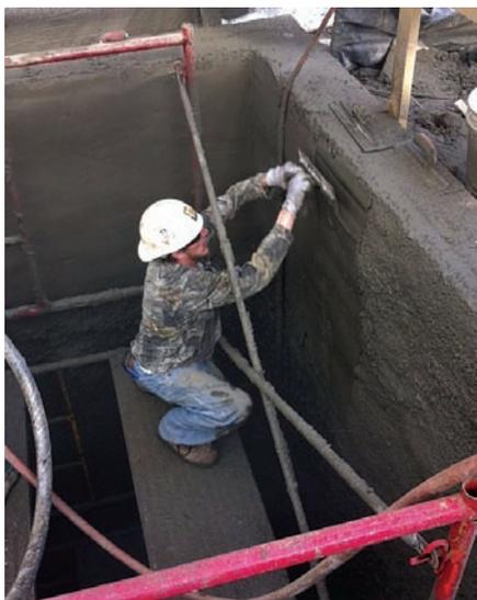
The crystalline waterproofing technology is non-toxic and contains no VOCs. This makes the crystalline material an ideal solution for applications in confined spaces.
